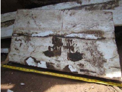
Below Grade Insulation St. Paul, MN
