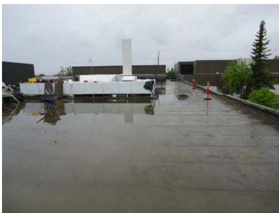
Roof A Wasilla, AK
